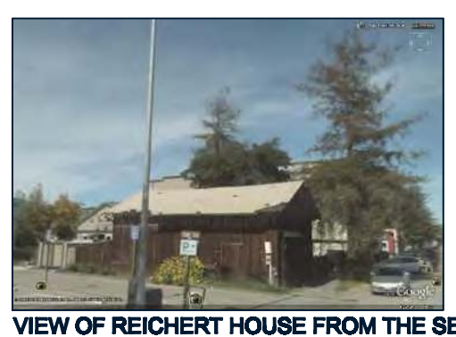
VIEW OF REICHERT HOUSE FROM THE SE
