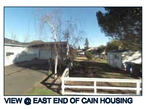
VIEW OF EAST END OF CAIN HOUSING
