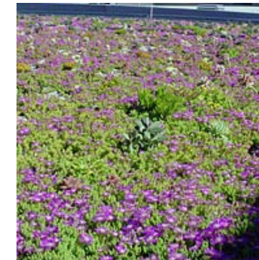
sedum for living roof
